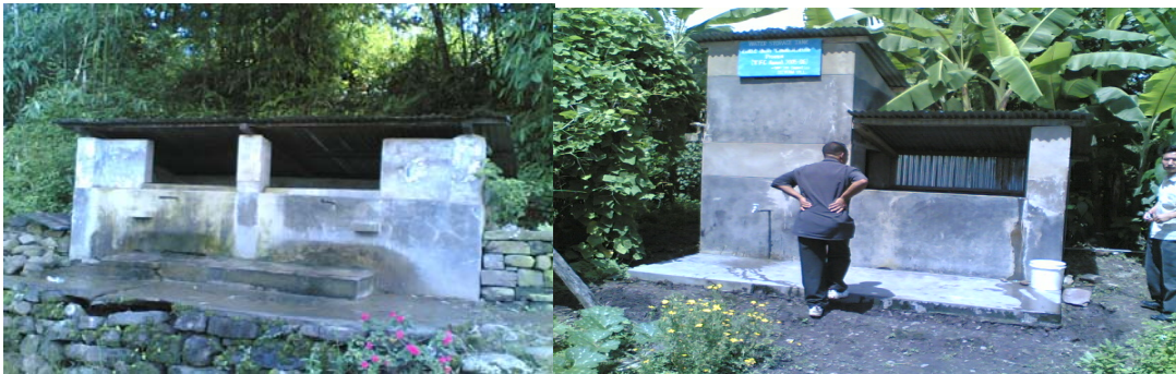
Water supply point provided by PHED
