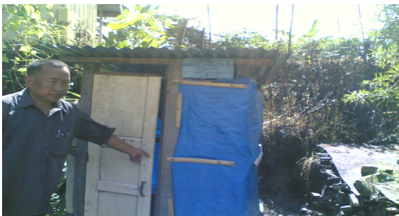
Toilet constructed with tin sheet and plastic
