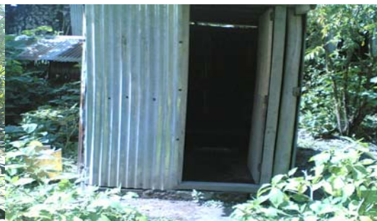
Toilet constructed with tin sheet
